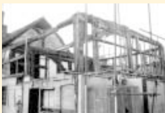
Wealden-house roof truss from Billingshurst, West Sussex. Dismantled 1968
