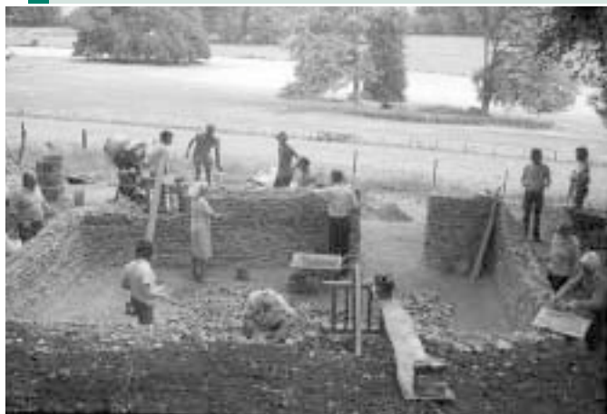
Archaeologists and volunteers building the conjectural flint walls of the 13th-century Hangleton cottage, based on the excavations at the structure's original site.
