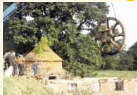
Dismantling under way, with the wheel being removed by a crane.
