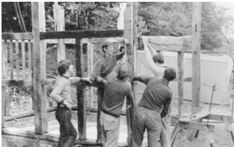
Boys from St Andrew's School, Worthing help Roger Champion re-erect the wheelhouse frame for Catherington treadwheel, 1970.
