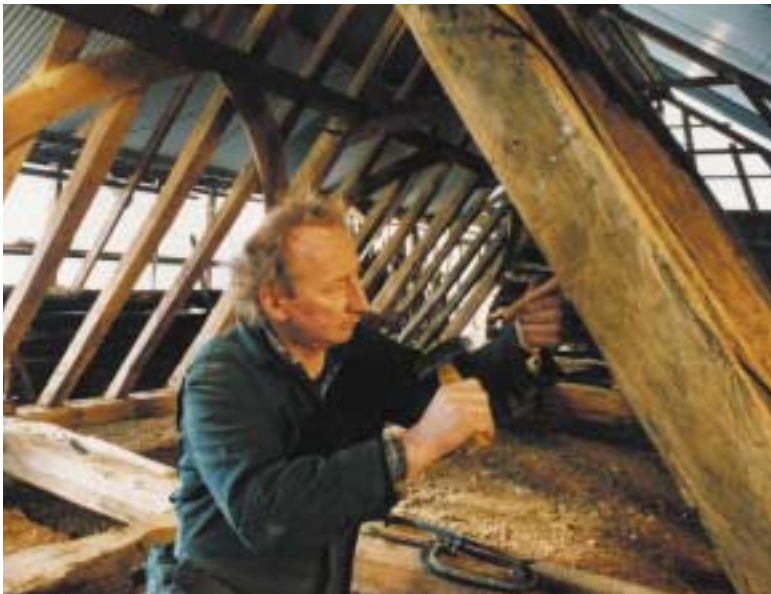
Repairing the roof of Longport farmhouse in the workshop at Charlton Barns.
