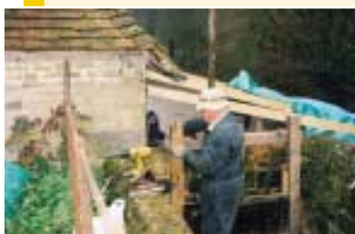
Robert Demaus dressing the mill's stones, a vital maintenance task to ensure the efficient production of flour, and below repairing the timber work at the mill leet.
