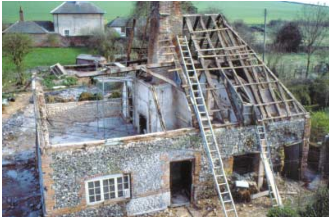
A high level view, looking south, during the process of removing the roof timbers.
