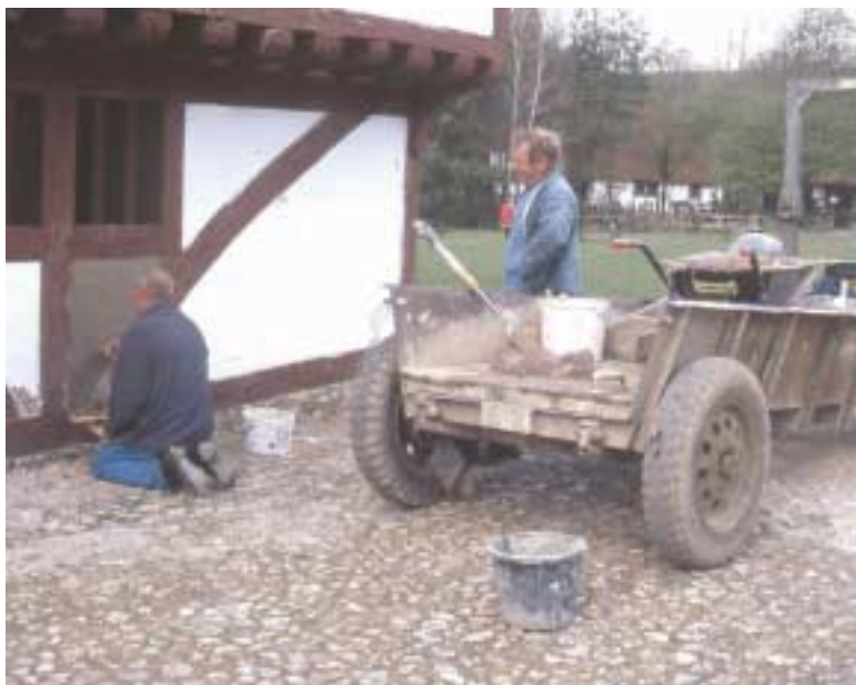
Daubing repairs under way at the house from North Cray, with Mick (left) and Ron Betsworth. Pete Betsworth, the first of the Betsworth brothers to be employed by the museum, is pictured on page 121.
