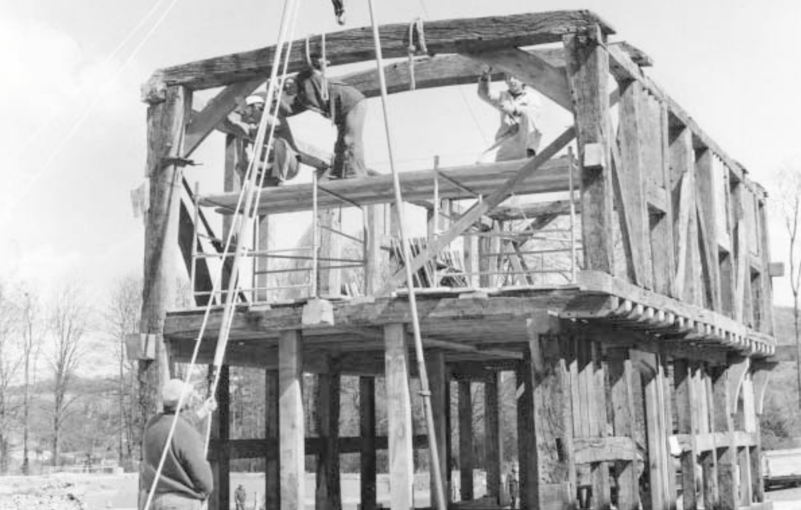
Re-erecting the framework of the upper hall from Crawley in 1978.
