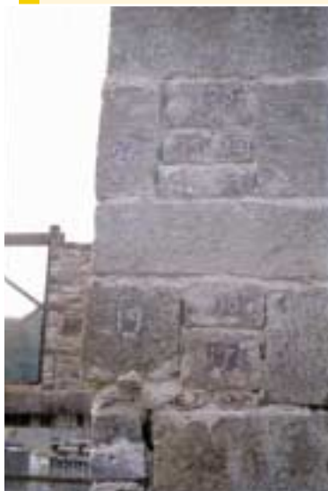
Major stones were numbered, to ensure their correct replacement during rebuilding.
