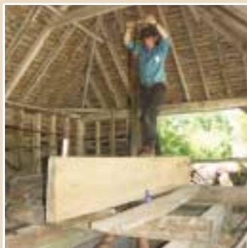
Jon Roberts pit-sawing – most timber for building was produced in this way until the 19th century.
