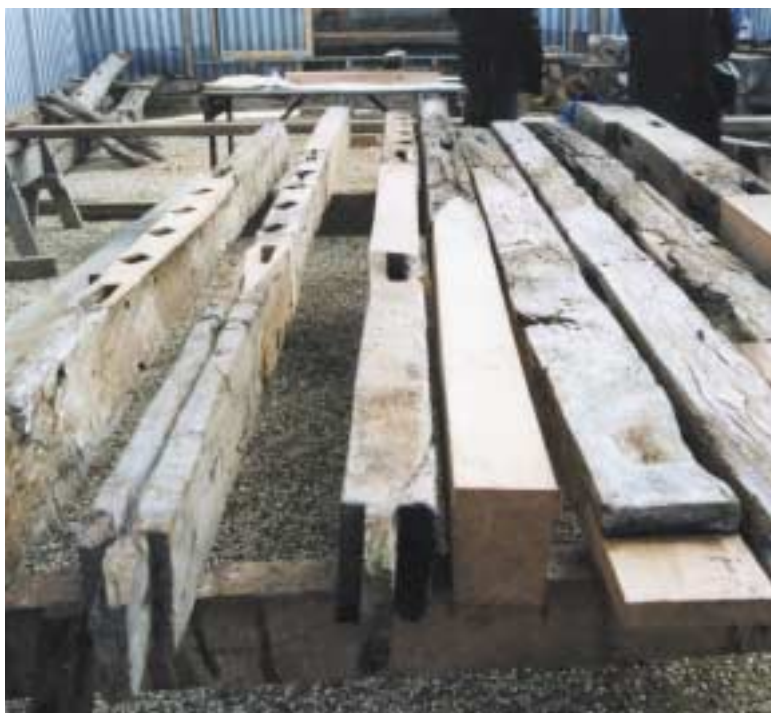
The timbers of Poplar Cottage laid out in an on-site workshop awaiting re-erection. Roger Champion’s repairs to the original timbers with new material can be clearly seen; the diamond shaped holes on the three timbers to the left will take the window mullions once re-erected.
