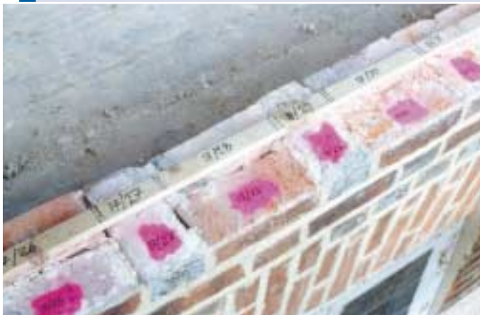
Above The number on top of each individual brick as they were dismantled from Longport farmhouse together with the corresponding batten, and below bricks and battens arranged in order at the museum, ready for re-building.
