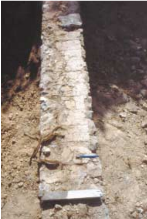
The joint lines of a row of bricks in a mortar bed revealed after removal of overlying flints, giving the position of a previously unsuspected window.
