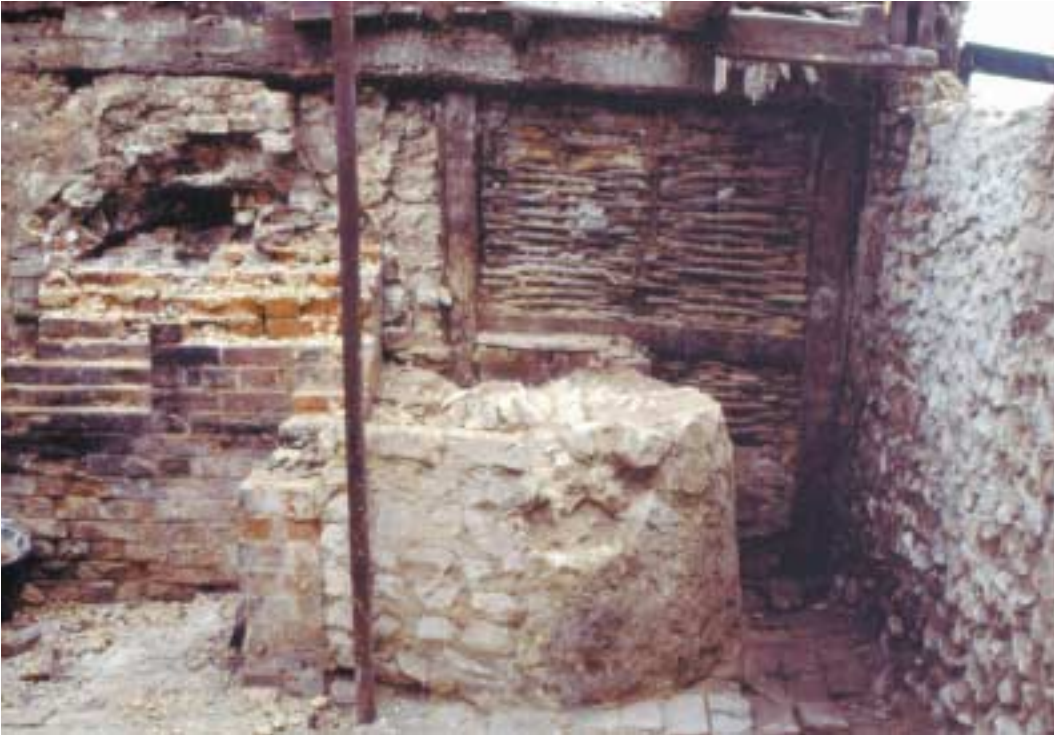
The chalk base of the oven built at the end of the 18th century. The dismantling revealed a succession of four ovens, of which this was the third; the arch of the original oven can be seen in the brickwork to the left.
