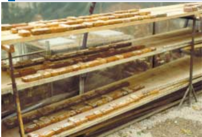
Above The number on top of each individual brick as they were dismantled from Longport farmhouse together with the corresponding batten, and below bricks and battens arranged in order at the museum, ready for re-building.
